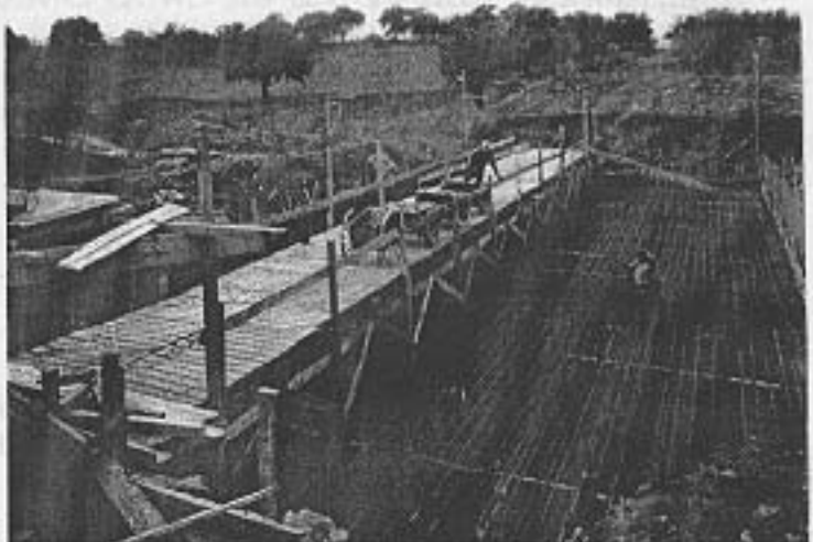
Construction of the 34th Street Bridge in the early 1930s.
